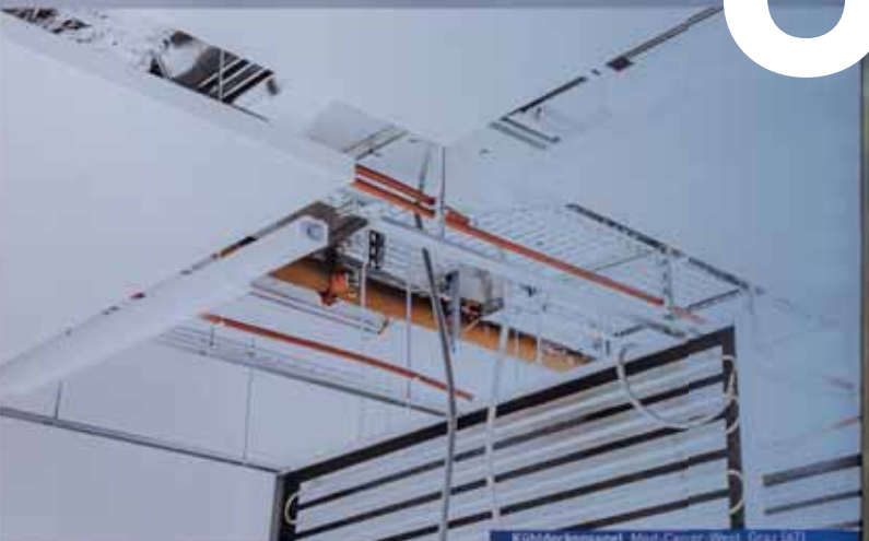
Kühldeckensystem Med-Center West, Graz (AT)
