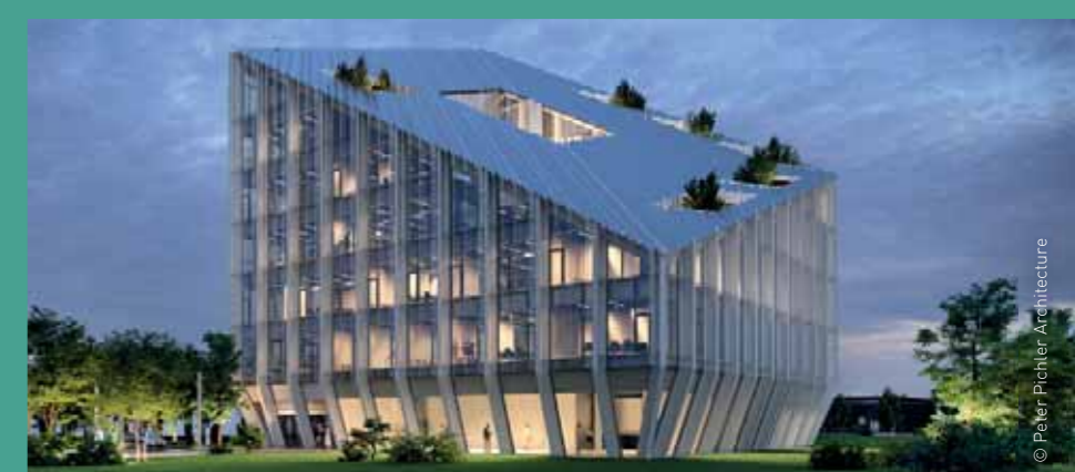
→ EVO Plant Bonfiglioli Headquarter Bologna, IT chladicí podhled
